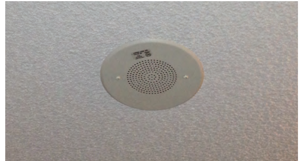
Fire Alarm Speaker – Do not disconnect
