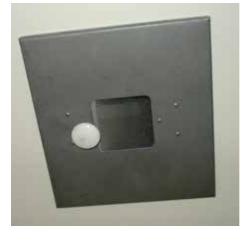
Laundry Room Lint Trap. Typically located above washer/dryer. Refer to Homeowners manual for suggested maintenance guidelines.
